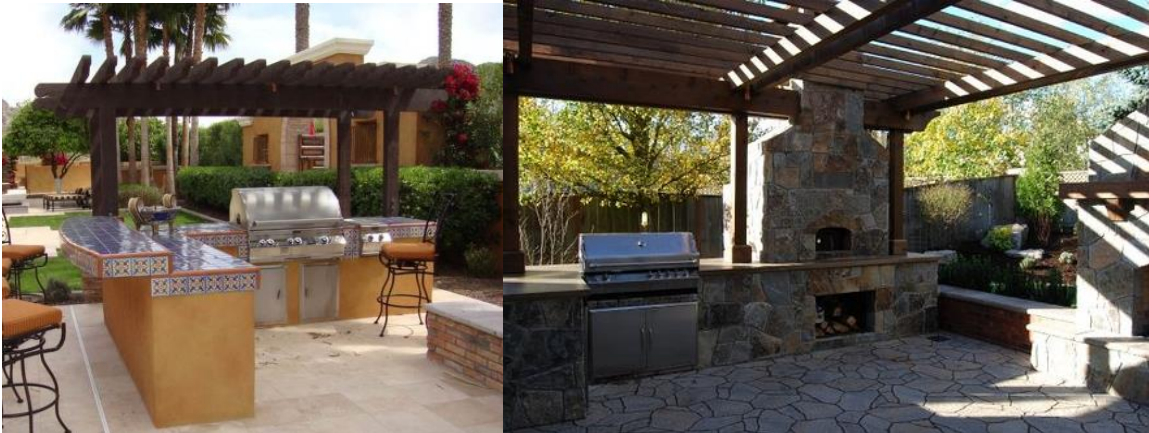
Figure 2: Pergolas, combustible structures
