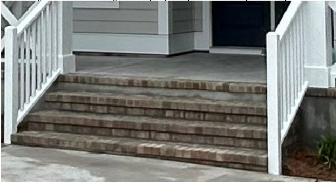
Figure 2: Stairs abutting cross-sloped paved patio or driveway – Close-up View
